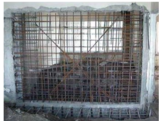
Figure 170 Adding new shear wall
