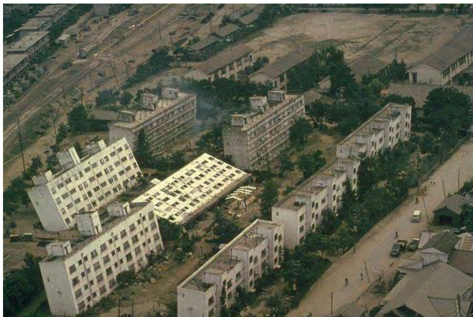
Figure 54 Buildings damaged due to soil liquefaction
